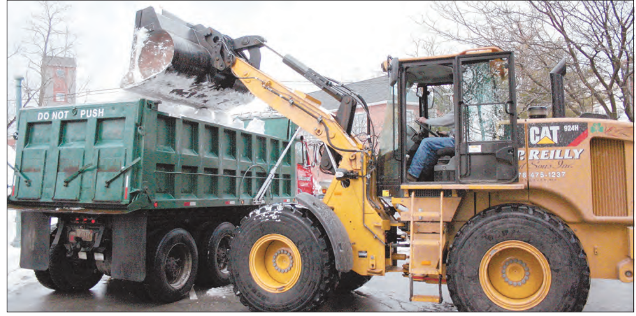
Mark Doherty, who works with private contractor F.P. Reilly & Sons, loads snow into a dump truck in the parking lot behind the Memorial Hall Library on Tuesday. Town crews and contractors worked around the clock this weekend and earlier this week to help the town remove around 27 inches of snow that dropped during last weekend's blizzard. DUSTIN LUCA/Staff Photo
