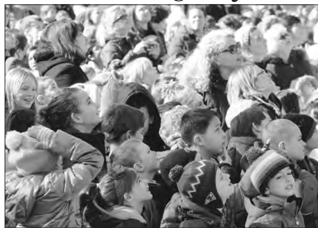
Students and teachers at Bancroft Elementary School look on in excitement as one of the final steel beams to be installed on the new Bancroft school is put in place. The beam was signed by teachers, students and town officials and installed as part of the last week's topping off ceremony at the school.
