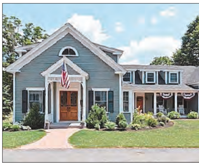
SYMPATHETIC ADDITION AWARD 154 ANDOVER ST. 1855 Hoffman-Murnane House, late Greek Revival Owners: Collen and Jeff Fuller Architect: Joanna Reck; contractor: Steve Dejardins Construction This home, which began as a German social club, was renovated and expanded in 2010. A large garage/barn and connector family room with master suite above was added and low-profile shed dormers to the existing structure created a second floor for children's bedrooms. The project retained existing historic details, resulting in a successful adaption for 21st century living.
