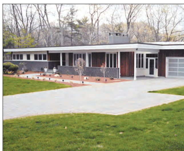
EXTERIOR PRESERVATION AWARD 18 ORIOLE DRIVE 1958 Blackman House, International style Owner: Tracy Goodman New renovations to the house have given it a fresh post-modern look, but allowed it to remain true to the original contemporary design reflective of the International style. The house maintains its rectilinear components of elongated rectangles of windows, horizontal and mixed sheathing materials and flat roof lines that seem to anchor it to the ground.
