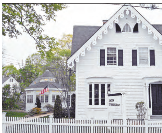
SYMPATHETIC ADDITION AWARD 34 ESSEX ST. 1845 Joseph Thompson Abbot House, Gothic Revival style Owners: Barry R. Finegold and William J. Dalton Architect: Gregory W. McIntosh, Lincoln Architects LLC Built by Jacob Chickering, this small Gothic Revival cottage is one of only three remaining homes in town to embrace this high style of architecture. A former parsonage, the house was converted into offices in 1983 and sold to the law firm of Barry R. Finegold and William J. Dalton in 2005. They razed a rear, 1980s addition and replaced it in 2012 with a two-story addition that successfully incorporates the Gothic Revival detail found in the original building.
