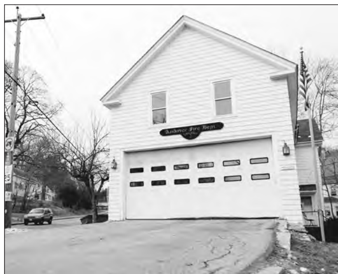
Replacement of the circa 1890 Ballardvale fire station at the intersection of Clark Road and Andover Street is among the priorities identified in Town Manager Reginald "Buzz" Stapeczynski's latest capital improvement plan. He is seeking $1.5 million next fiscal year to buy land and design a new station.
