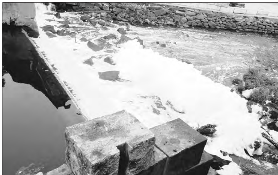
Foam built up at the base of the Ballardvale dam on the Shawsheen River last week. The foam was caused by fire retardant used on a plane crash at Hanscom Field earlier this month that killed seven people.
