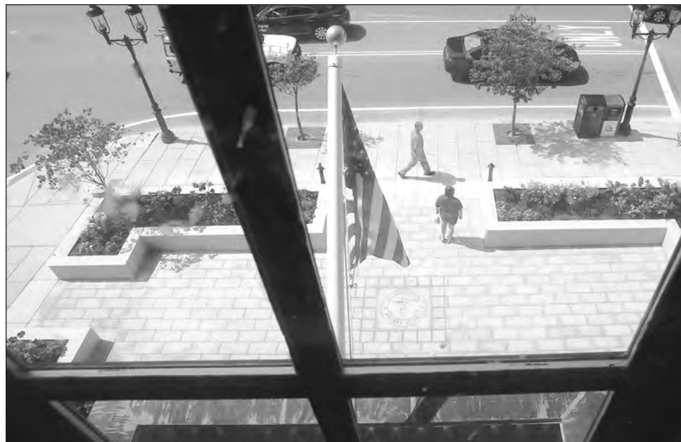
MARY SCHWALM/Staff photos The view of the renovations in front of Old Town Hall in downtown Andover looking down from inside the historic structure. A town seal, below the American flag, is inscribed on one of the newly installed sidewalk stones.
