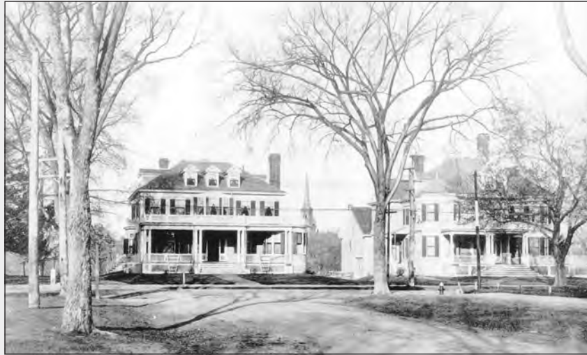
The homes at 93 Main St., left, and 89 Main St., were purchased in 1961 by Lincoln Giles, who built around the houses and named the area Olde Andover Village. The Andover Historical Society will highlight the history of Main Street on its Sunday afternoon tour.
