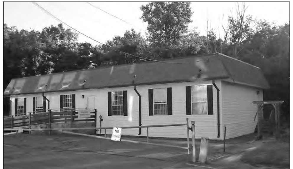
The modular classrooms at Shawsheen School are set to be demolished by the end of the month.
