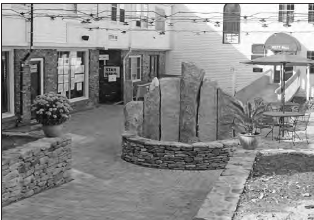
STAFF PHOTO TERRY DATE A soon-to-be finished fountain at Andover Village Square off Main Street. It will include a pair of opposites -- fire and water elements.
