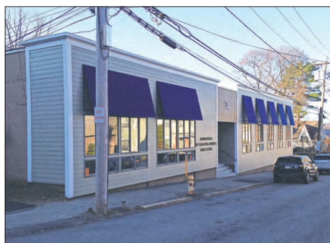
Here is 26 Essex St. after its renovation.
