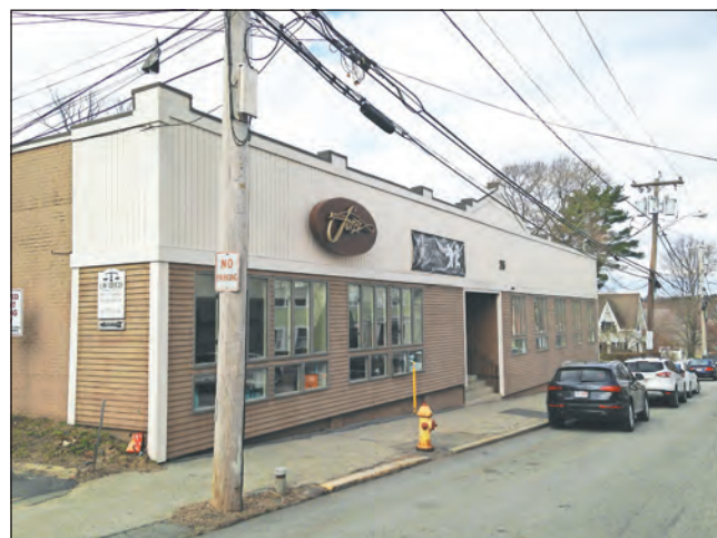
Here is the building at 26 Essex St. before its renovation.
