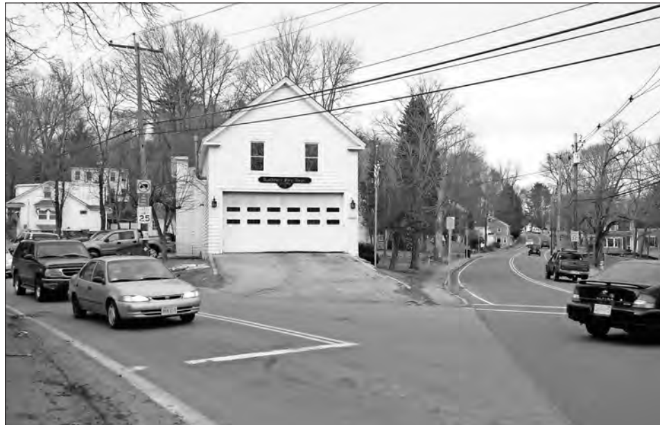
The Ballardvale fire station is at a difficult intersection. If the truck needs to make a left turn out of the garage it has to do a multi-point turn, delaying response time and creating a traffic jam.
