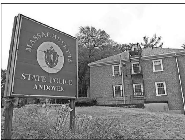
TIM JEAN/Staff photo Suspects arrested by the state police are currently being booked at the Andover Police Department while the state police barracks on Route 125 undergoes renovations.
