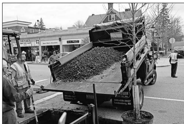
Members of Andover's Department of Municipal Services dump special soil created by Cornell University into the tree pit.
