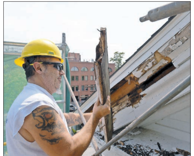
Noel Viana removes the old rotten trim of the roof.
