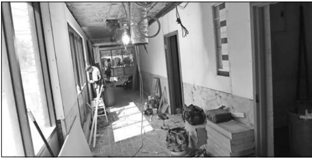
Carpenters from Marceau construction install drywall and tiles.
