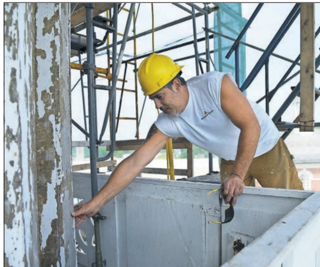
Noel Viana inspects the wooden trim of the church steeple.
