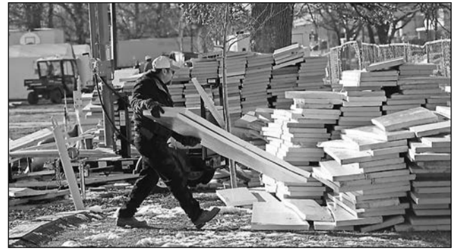
Workers move insulation brought in for the bottom of trailers.
