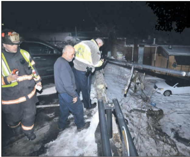
From left, Andover Fire Lt. Tom Kennedy, an unidentified man from Elm Street Towing and Andover police officer inspect damage to the wall and guard rail after the vehicle is removed.
