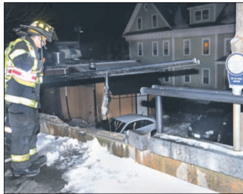
Andover firefighter inspects the damage to the wall and guard rail after the vehicle is removed by Elm Street Towing.
