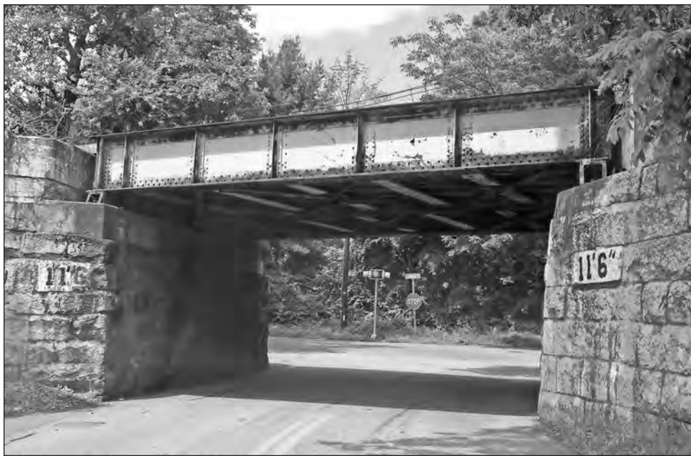
Horn Bridge on Central Street.
