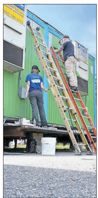
John Hancock employees paint a Habitat for Humanity home in Andover.
